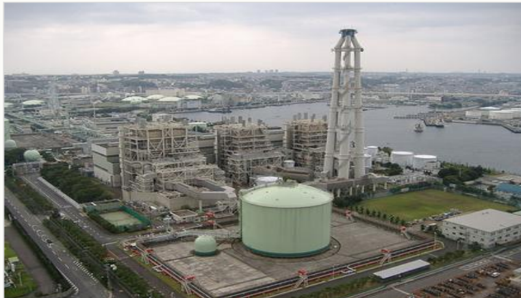
A TEPCO plant in Yokohama
